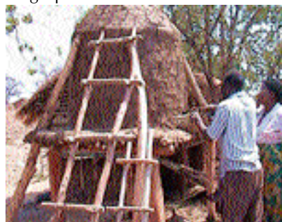
This improved traditional grain store is able to keep grain bug-free and safe for six months or more
